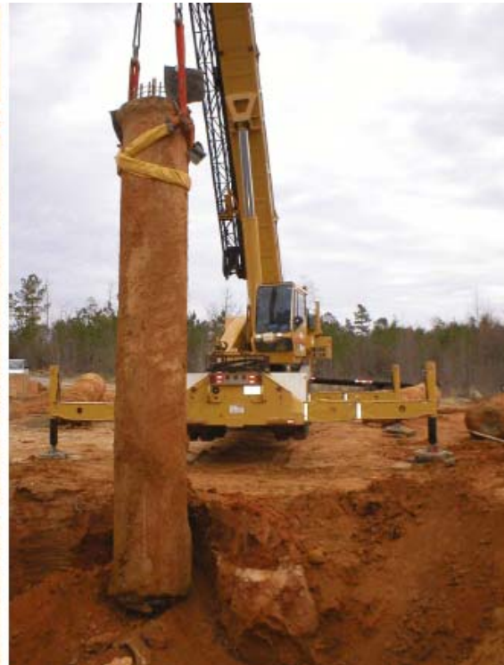
Drilled shaft exhumed after testing to verify grout distribution.
