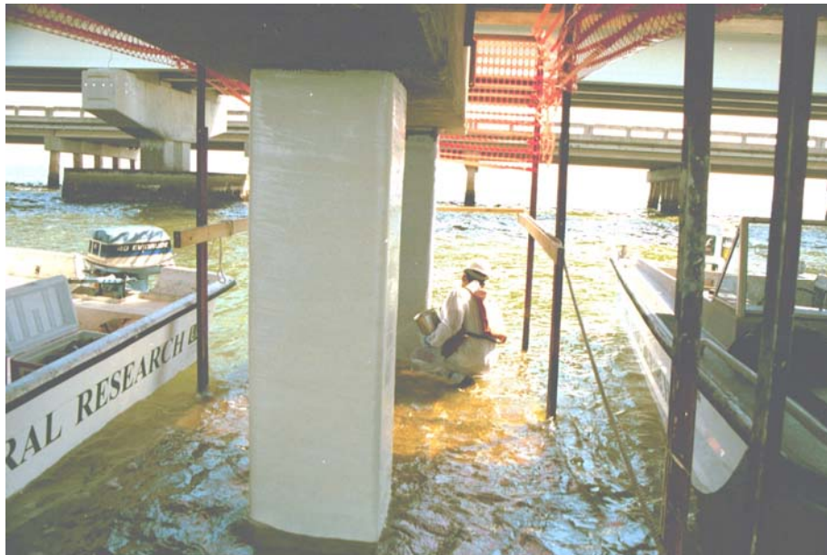
Repaired piling receiving the finishing touches.
