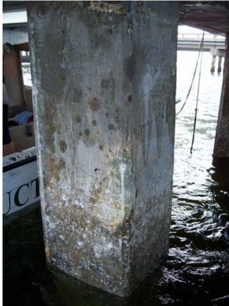
Pile ready to be repaired.
