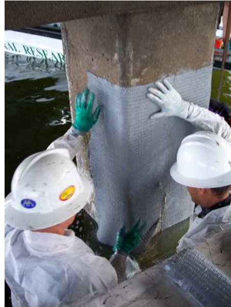
Application of fiber reinforce polymers.
