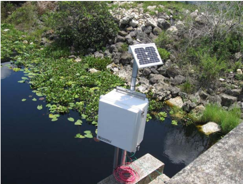
Corrosion monitoring, Everglades
