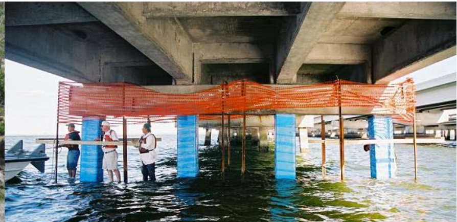
FRP Bridge Repair, Tampa
