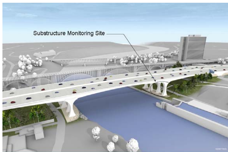
Rendering of the new I-35 bridge showing USF/FHWA/FGE monitoring site.
